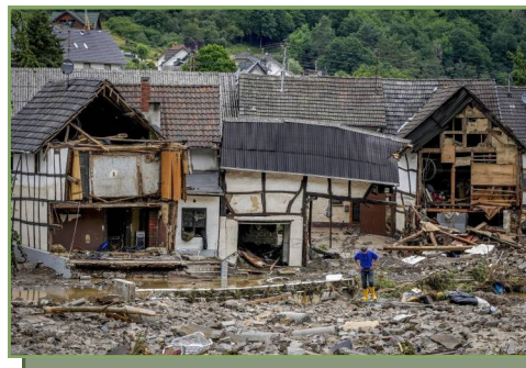
A photo from the neighboring village of Schuld that has been completely washed away
